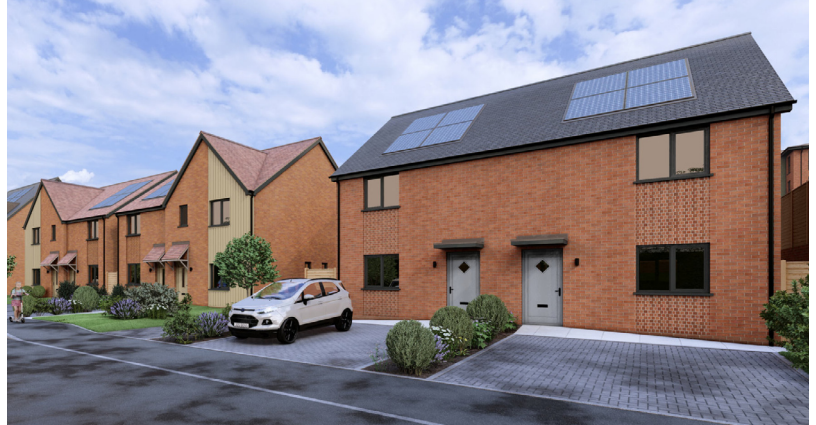
View of new houses along Valley Road (from where existing Valley Road garages are)
